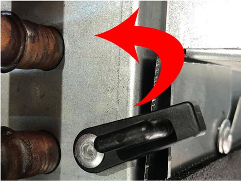
Step 2: Visually Locate Drain Pan Retention Studs.
