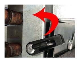
Step 2: Visually Locate Drain Pan Retention Studs.
